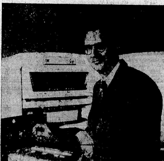
$5,000 FOR AUTOMATIC DEFROSTING. Graham S. McCloy thought housewives should be freed of the messy job of refrigerator defrosting. So he developed the "Frost-Free" refrigerator which defrosts itself automatically and with practically no rise in temperature inside the refrigerator. No thick frost layer ever builds up, and foods stay in perfect condition. The invention earned him a $5,000 award, and promotion to Section Manager.
